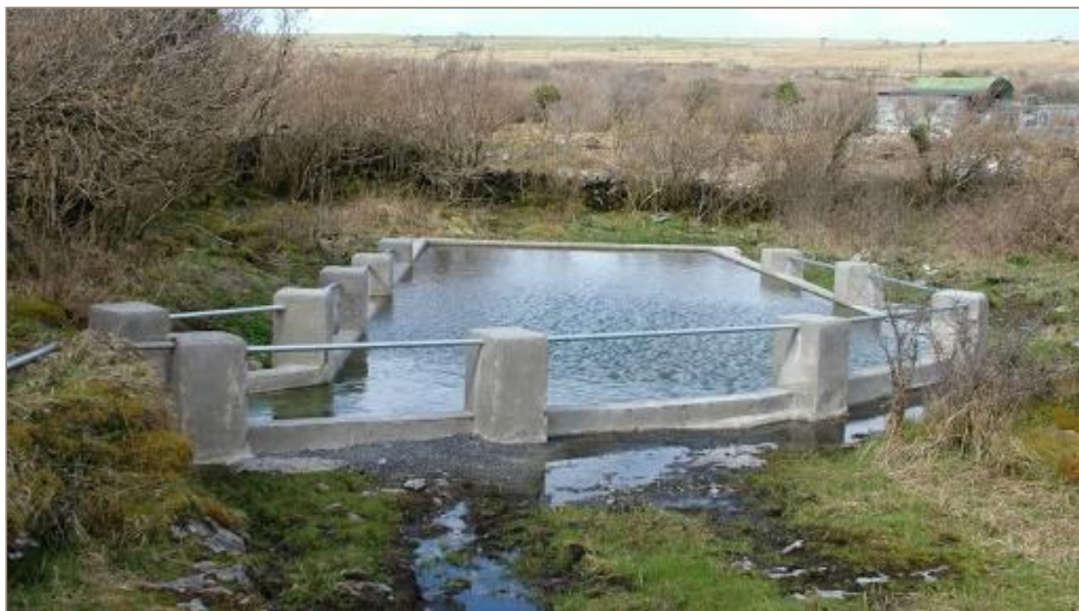
Figure 6.6: Example of a water storage tank
